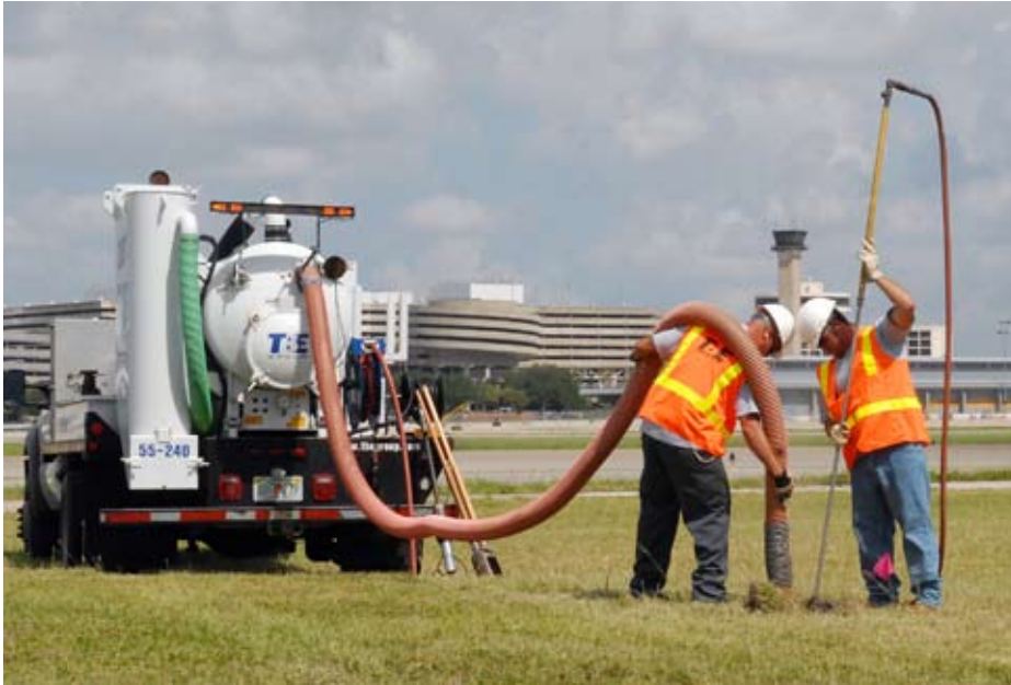
Vacuum excavation is used to locate the exact horizontal and vertical location of buried utility.
