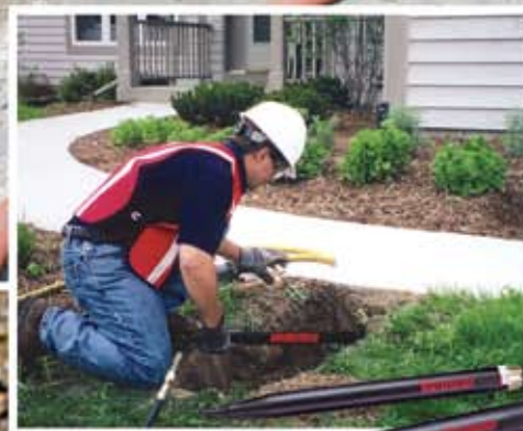
HammerHead® Mole Pneumatic Piercing Tools Sizes: 1-3/4" to 23"
