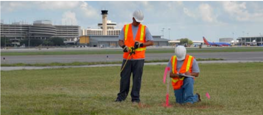
Test hole data provides useful information for design decisions.
